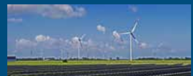
Photovoltaic and wind power plants.
